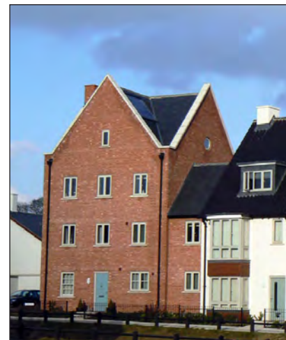
A notable corner expressed through scale, height and roof form of the house
