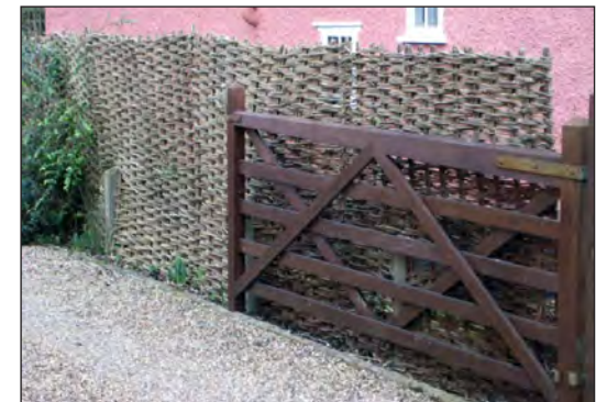
A hurdle fence in a rural setting provides a rustic boundary between plots where this is visible from the street
