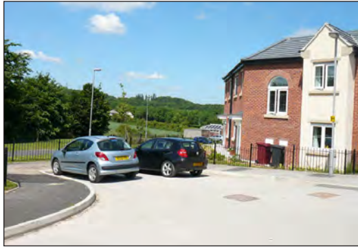
Cars parked within a turning head cause an obstruction to service vehicles needing to turn
