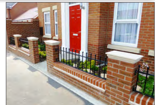
Modest brick walls and railings reflect their context and provide defensible space to small front gardens
