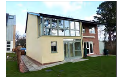
A large window for solar gain and a deep overhang and canopy for shade
