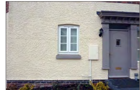
Where meter boxes can only be positioned on a prominent elevation this should be finished in a colour to complement the background material
