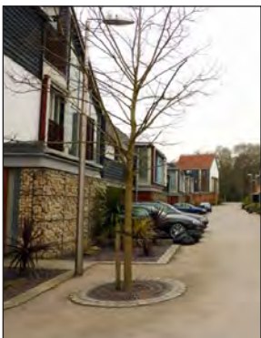
A poorly located tree in relation to the adjoining street lamp will block its light
