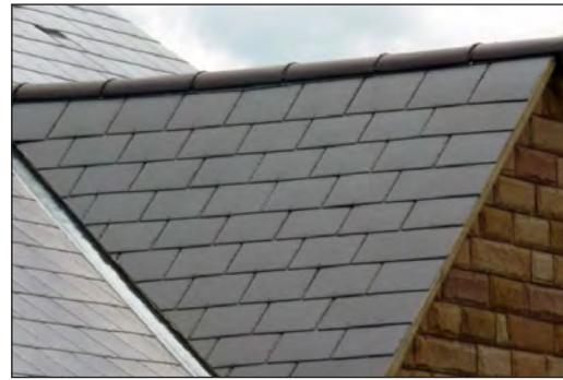
Slate roof with a thin leading edge profile provides a high quality finish
