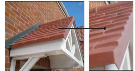
Above: Mass produced materials like moulded glass reinforced plastic (GRP) are inauthentic, appear crude and undermine the quality of the development
