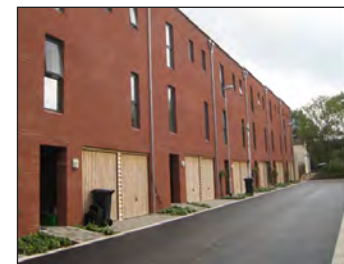
Largely blank ground floor elevations deaden the street scene and limit surveillance of public areas
