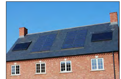
Solar panels reduce energy demand and lower running costs but need to face close to south and lie at 45° for maximum efficiency
