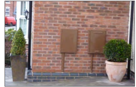
Meter boxes carefully located on a flank wall and coloured to complement the brick tone
