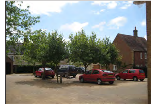
An attractive parking court enhanced by trees and overlooking from adjacent houses
