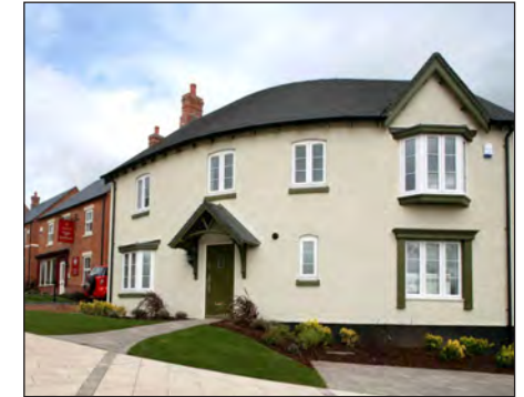
A house type designed to handle a corner and address both frontages (Davidsons Group Ltd)
