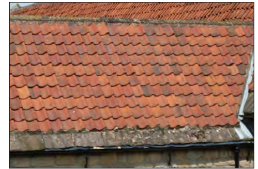
Clay pan tiles and stone slates in a rural context
