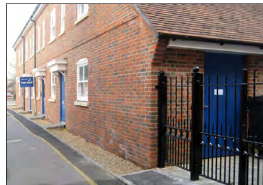
Above: Communal bin storage integrated into a lean-to, behind a secure gate and with external access only
