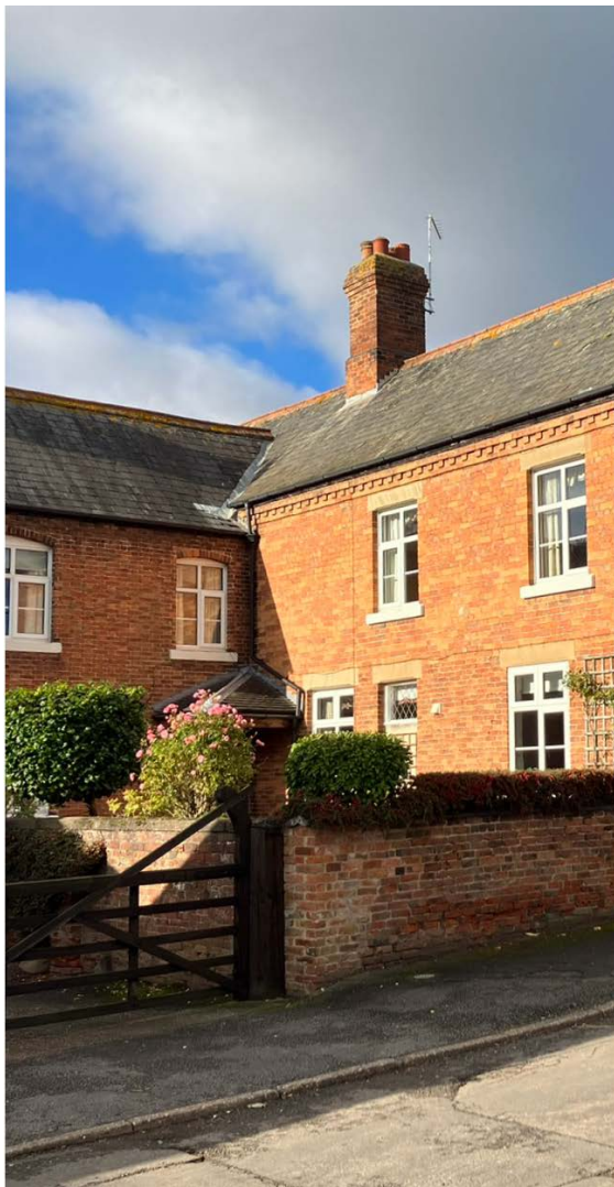
Photo 1 The layout of many traditional buildings in Elkesley creates a courtyard space
