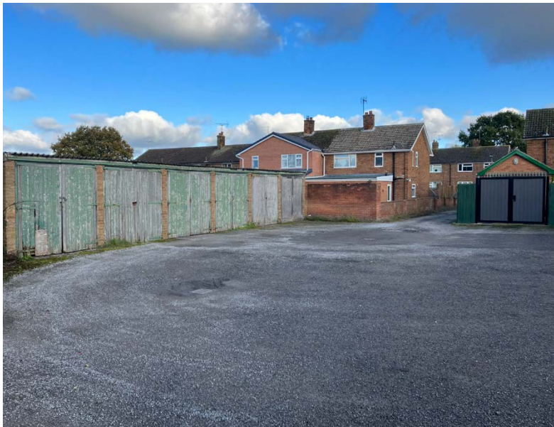
Photo 15 Site 2 Garage site off Lawnwood Avenue
