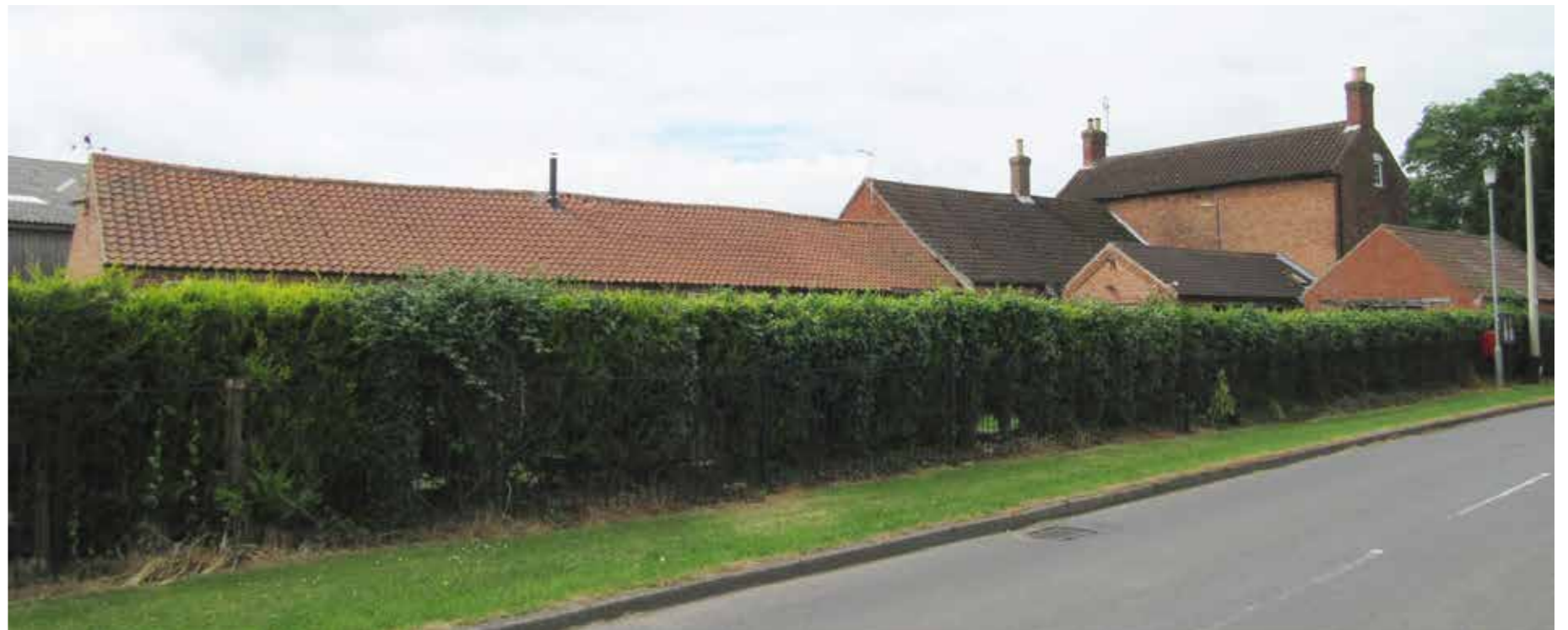
Fig 102: The original Manor Farm buildings have a much more harmonious relationship with the surrounding village setting, having retained a boundary of hedgerow planting, and presenting a more familiar and locally distinct domestic scale and appearance.
