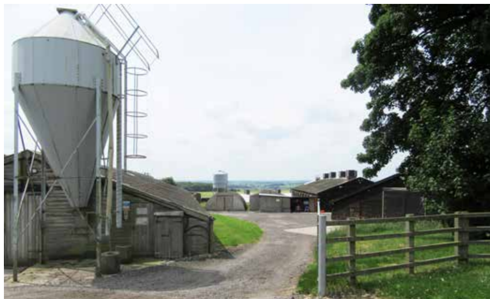
Fig 26: Located on the site of the former Grove Hall, Bodway Poultry Farm is the most sizeable non-residential use in the village.
