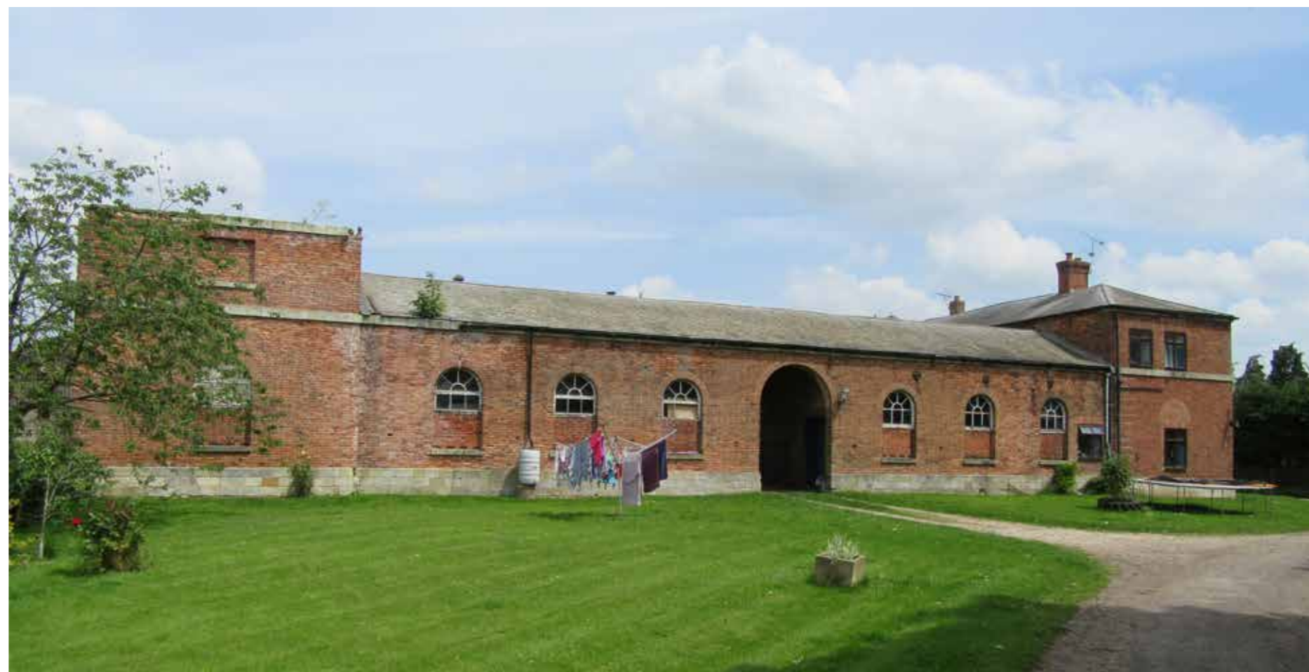
Fig 72: Though partially derelict and in a slight state of disrepair, Grove Hall Stables remains a captivating piece of locally distinct architecture, representing one of the key remaining structures with direct links to the former Grove Hall estate.
