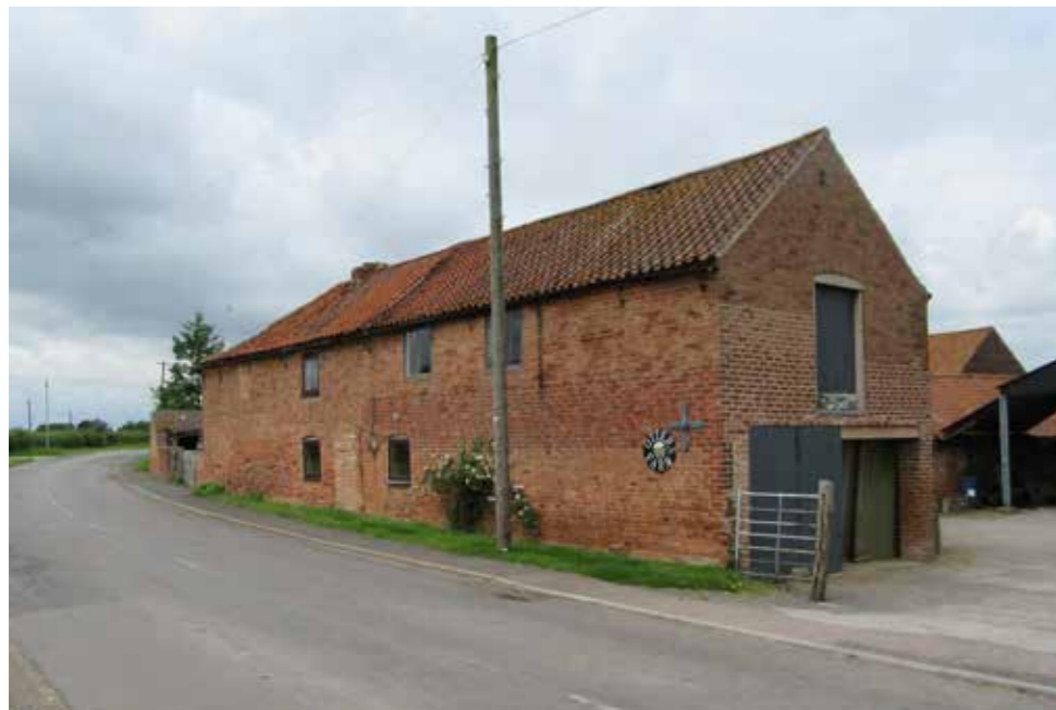
Fig 114: The charming barn building at Otters Farm presents a unique and locally distinct frontage along Main Street.
