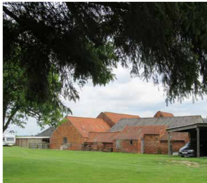
Fig 115: Set back from Main Street are further vernacular buildings associated with Otters Farm, all presenting the same rich red brick walling and pitched clay pantile roofs
