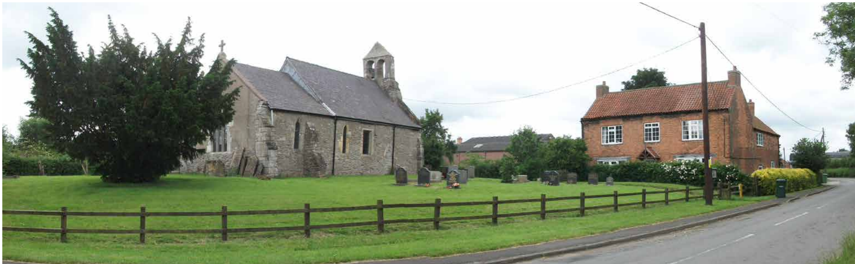
Fig 123: Views towards St Peter's are pleasingly open, allowing a full appreciation of the church's form and fabric from Main Street whilst simultaneously enhancing the character of the surrounding townscape. The positive influence of Church Cottage is also nicely illustrated within this view, its attractive red brick facade and pantile roof contrasting pleasingly with the church's various tones of grey, and also working with the church to frame the churchyard setting and a create a delightfully composed and memorable piece of townscape.
