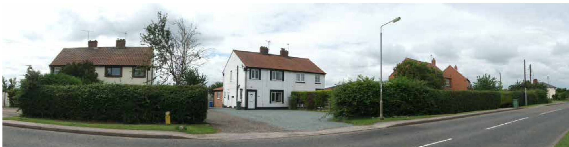
Fig 96: Semi-detached dwellings sit back from Laneham Road within long narrow plots and behind garden hedgerows.
