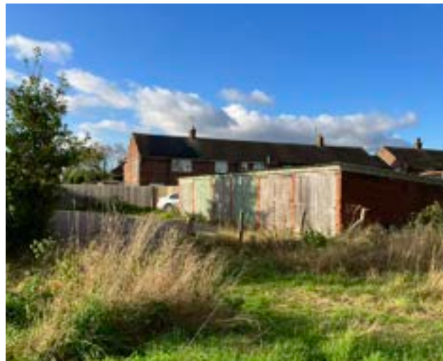
Figure 72: Underutilised garage sites on both Headland and Lawnwood Avenues could also provide an opportunity for community growing spaces.
