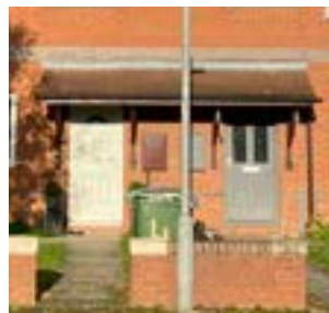
Doors with angled, tiled canopy
