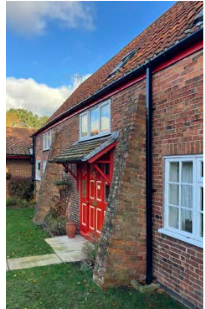
Figure 01: A historic dwelling in Elkesley, featuring an L-shaped plan at 90 degrees to the street, brick buttresses and a tiled door canopy.
