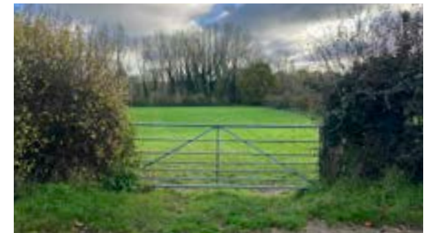
Figure 81: Land adjacent to Brough Lane often floods in times of heavy rain. New development within the Poulter Valley should be avoided.
