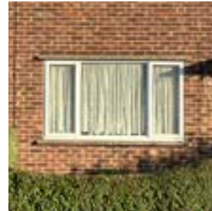
Casement windows with stone lintels
