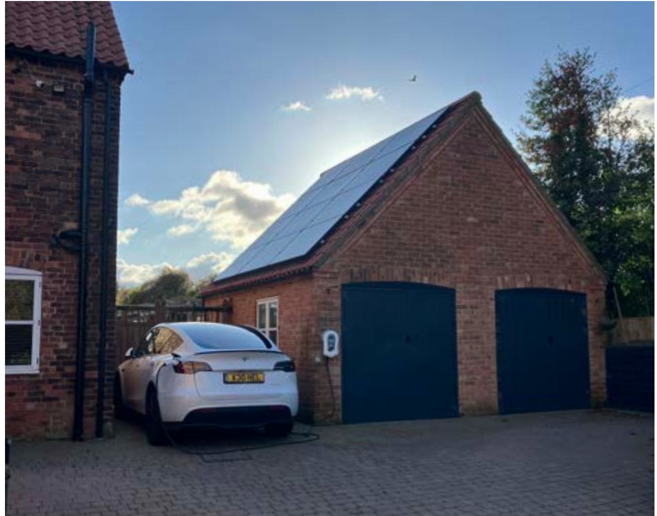
Figure 83: Solar panels and an EV charging point integrated within a garage in Elkesley Village.
