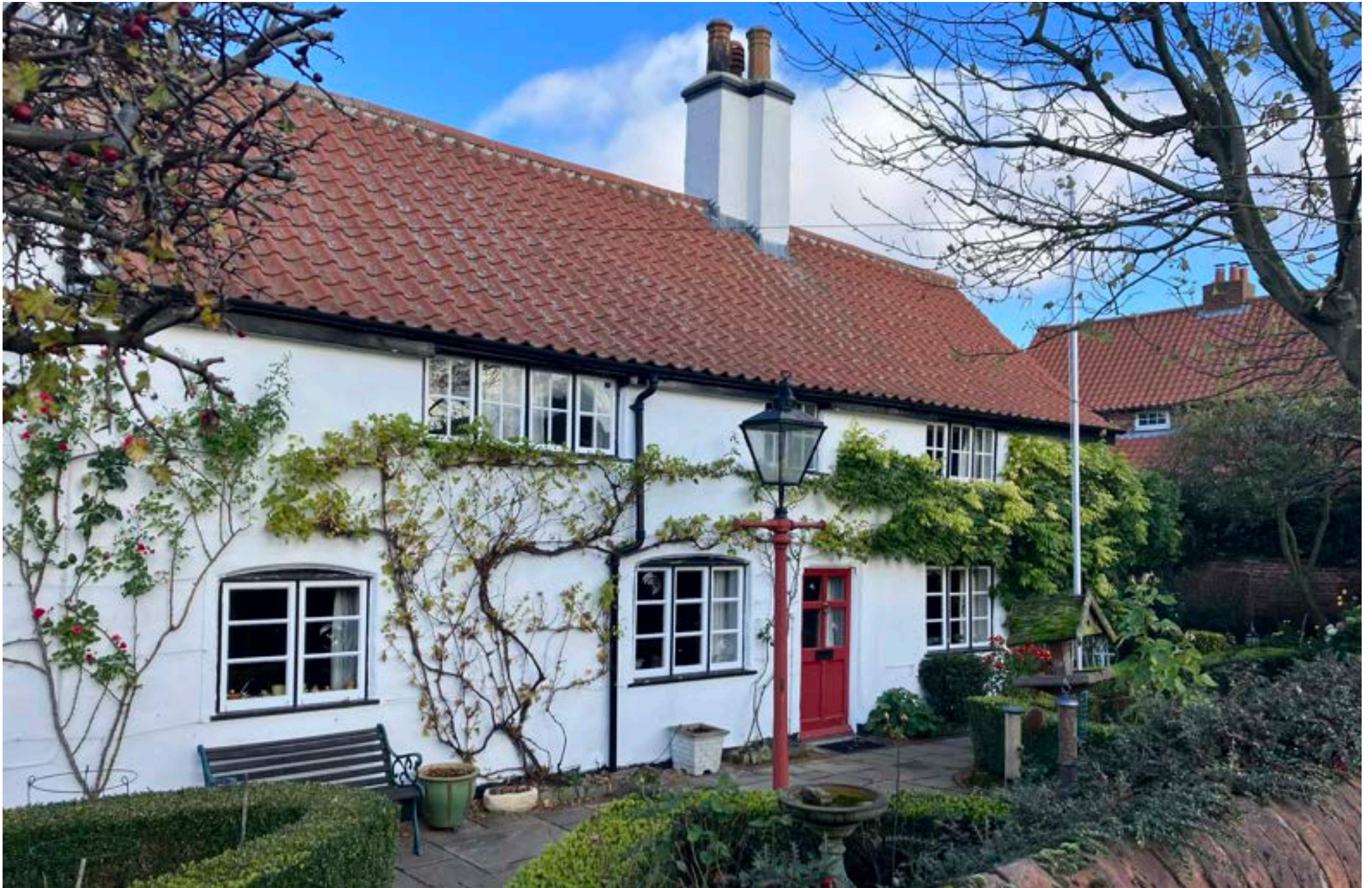
Figure 03: Meadow Farmhouse, a Grade II Listed building on High Street. Featuring a white cement render, red pantiles, segmental arches on ground floor openings and casement windows with glazing bars. A low red brick wall creates a boundary with the street.
