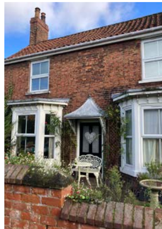
Figure 44: A home in Elkesley, set back from the pavement with a small front garden creating a relationship with the street. Features red brick, a red pantile roof and bay windows. New development should respect and respond to traditional character features such as these.
