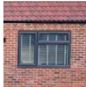
Casement windows with grey frames
