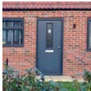
Partly glazed door set within main facade
