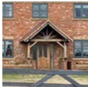
Timber framed porch
