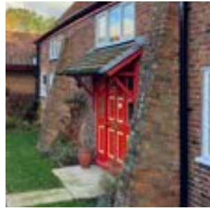
Wood panelled door with surround and canopy
