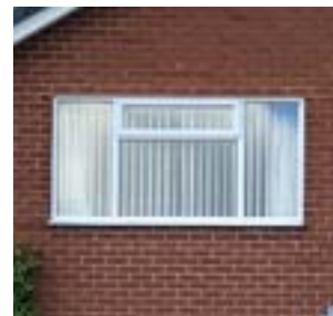
Casement windows with white frames
