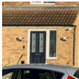
Partly glazed door set within projecting porch
