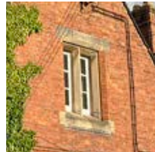
Stone mullion windows with stone lintels
