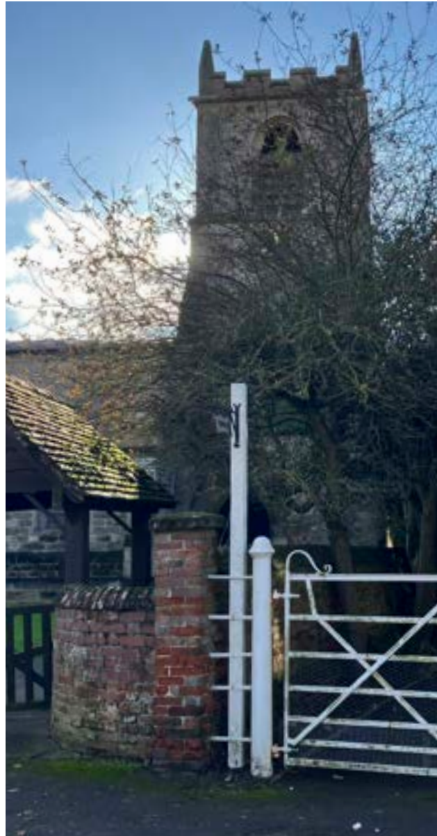
Figure 10: The Grade I Listed St. Giles Church was constructed circa 1300 and sits at the heart of the village.
