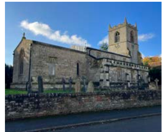
Figure 45: The Grade I Listed Church of St. Giles, located on High Street.
