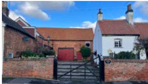
Figure 50: The Grade II Listed Meadow Farmhouse, an example of a cluster of converted farmbuildings with an L-shaped arrangement, forming a courtyard.
