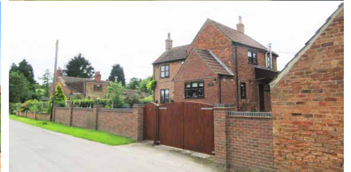
Fig 166 - 167: The Holding sits to the immediate north of The Homestead, where its sizeable and distinct parallel roofed profile is relatively exposed in views along Greenspotts Lane. Through displaying a materials palette that is in keeping with the surrounding area, a lack of greenery combined with the imposing and formal nature of its boundary walling and driveway entrance give the dwelling a more suburban appearance that is somewhat out of sync with the wider rural character.
