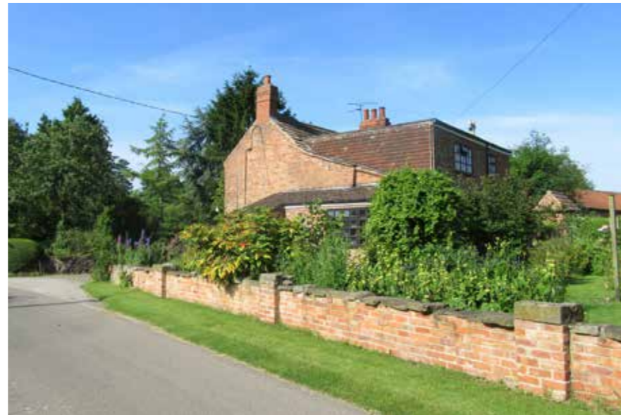
Fig 164 and 165: The Homestead is a 19th century cottage whose linear form runs perpendicular with Greenspotts Lane. Despite some alterations and additions, including a large dormer on the original rear projection, the building still retains much of its original charm and character, which is complemented by a diversity of garden planting and a low-lying red brick, stone-capped wall.
