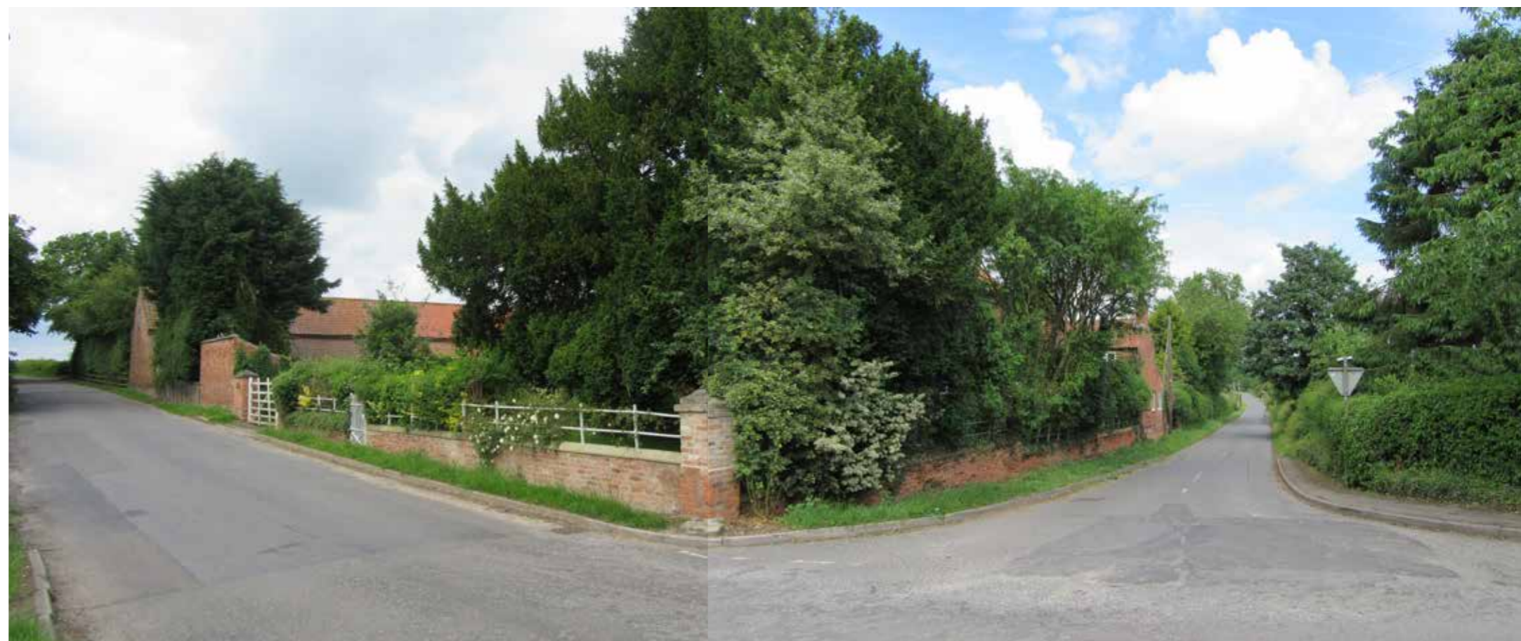
Fig 279: The eastern corner of the junction of Main Street and Yew Tree Road is occupied by the most historic structures of Grange Farm, whose rich red fabric peeks out from behind dense tree planting, which is in turn bounded by particularly handsome stone capped, red brick walling that also incorporates simple yet aesthetically pleasing white painted, cast iron railings.
