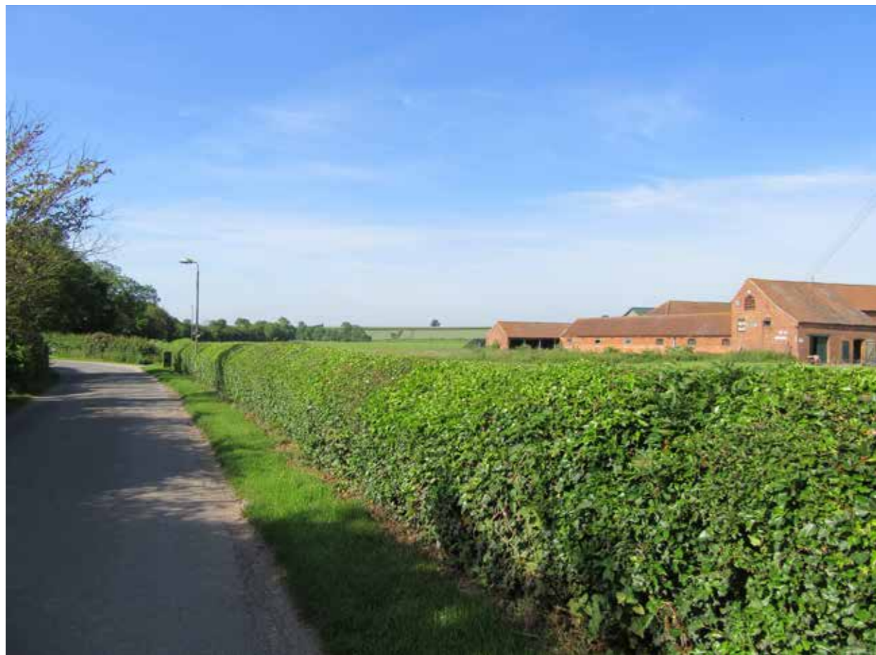
Fig 155 and 156: The cluster of red brick outbuildings at Headon Manor Farm includes a threshing barn, stables, cart sheds and animal sheds, and a dovecote with a distinct east facing gable incorporating arched flietholes. This attractive grouping of agricultural buildings has a distinct roof profile, and is complimented by a backdrop of open landscaped topped by big, sweeping skies.
