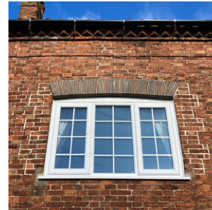
Casement windows with glazing bars and curved lintels
