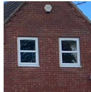
Casement windows with white frames
