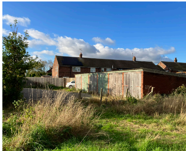
Figure 72: Underutilised garage sites on both Headland and Lawnwood Avenues could also provide an opportunity for community growing spaces.
