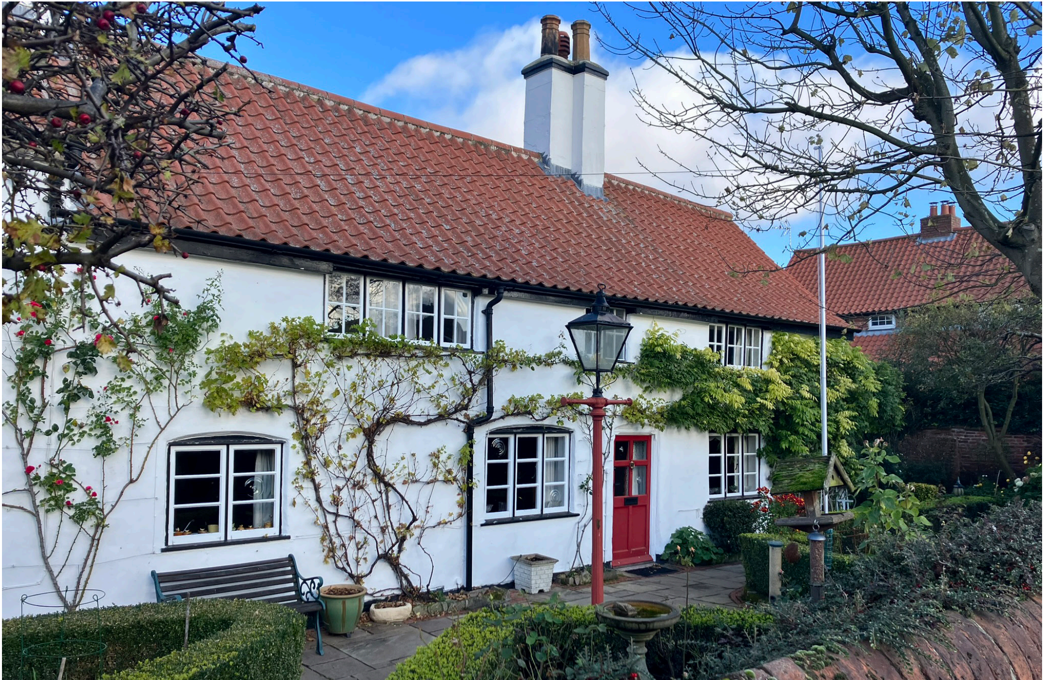
Figure 03: Meadow Farmhouse, a Grade II Listed building on High Street. Featuring a white render, red pantiles, segmental arches on ground floor openings and casement windows with glazing bars. A low red brick wall creates a boundary with the street.
