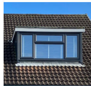
Casement windows within a dormer
