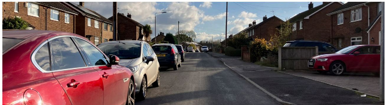
Figure 66: Off-plot parking is not acceptable as it negatively impacts the streetscene and narrows road widths, exacerbating congestion and reducing traffic flow.
