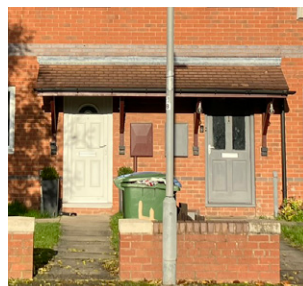
Doors with angled, tiled canopy
