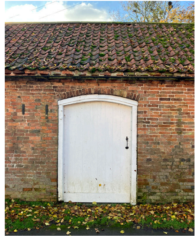
Figure 51: Grade II Listed structures at Portland Farm which front directly onto the pavement, featuring curved door lintel and dentil brickwork along eaves.
