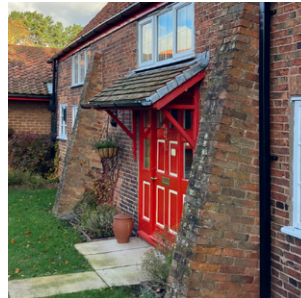
Wood panelled door with surround and canopy
