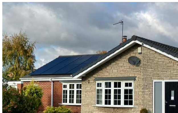
Figure 84: Solar panels in use across different styles of roofscape in Elkesley.
