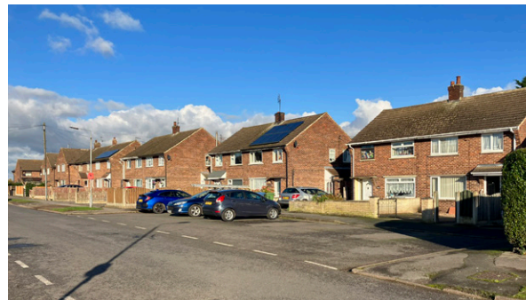
Figure 80: The drainage on Headland Avenue is often overwhelmed in times of heavy rain.
