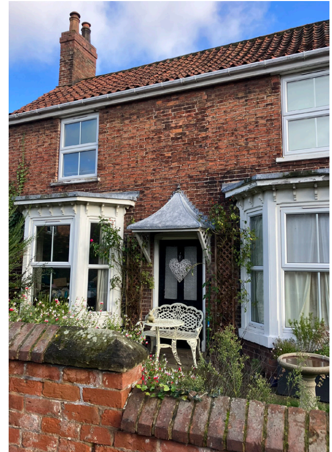
Figure 44: A home in Elkesley, set back from the pavement with a small front garden creating a relationship with the street. Features red brick, a red pantile roof and bay windows. New development should respect and respond to traditional character features such as these.
