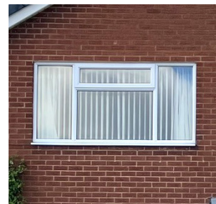
Casement windows with white frames
