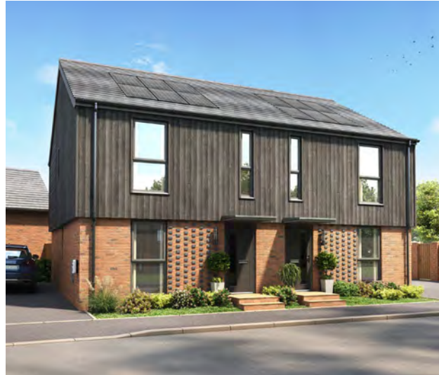
Figure 74: Carbon negative affordable homes in Derbyshire.
