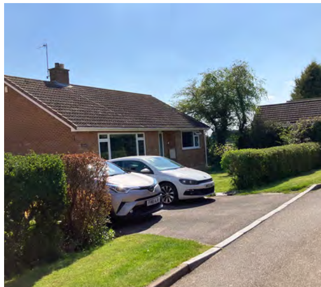
Figure 63: Front of property parking with hedgerow screening.
