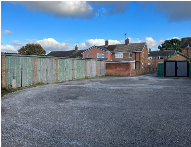
Photo 15 Site 2 Garage site off Lawnwood Avenue
