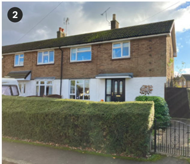
Figure 07: Mid-20th century homes face the site on its southern boundary. These are two-storey with low hedgerow boundaries.
