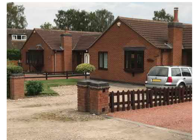
Brown PVC windows with lead came.
