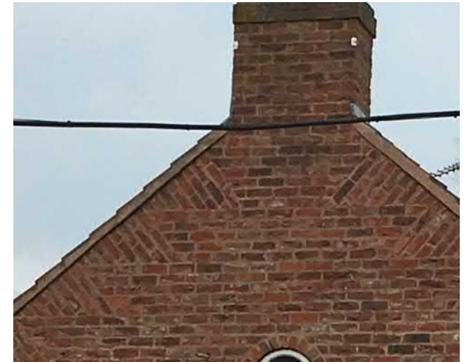
Brick detailing along the roof line of a gable end.
