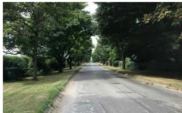
4. Daneshill Road looking west.
