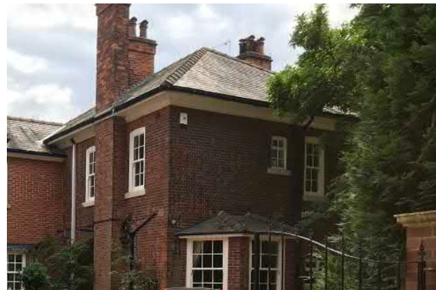
Tall chimneys serving multiple rooms within a house
