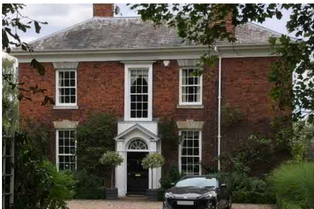
The Elms. Constructed with a red brick flemish bond and a slate hipped roof with a white painted cornice, symmetrical window alignment and a centrally positioned front door.
