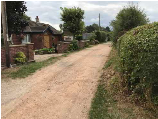
Little Top Lane lacks formal paving or road surfacing
