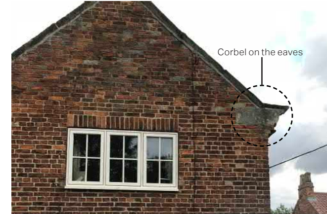
A house with a corbel on the eaves
