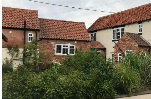
Roofing covered with red pantiles
