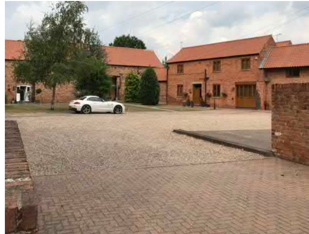
Highfield Farm barn conversion with parking courtyard, and gable roofs covered with red pantiles
