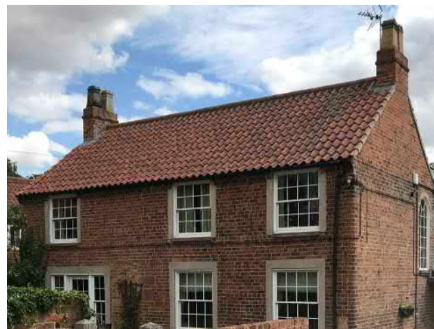
Chimneys positioned on the gable ends of a dwelling
