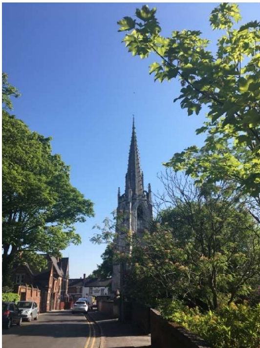
KV2: Looking north east along Rectory Road to St Michael the Archangel – a key landmark building Grade 2*
