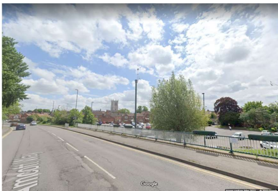
KV5: Looking south east across Amcott Way and Churchgate Car park long view to St Swithun's
