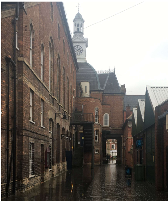
KV12: Looking north along Town Hall Yard
