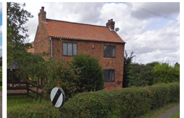
Fig 47: Two-storey detached dwellings with pitched pantile roofs accommodating chimneys and red brick walling are the most locally distinct building typology seen in Cottam.
