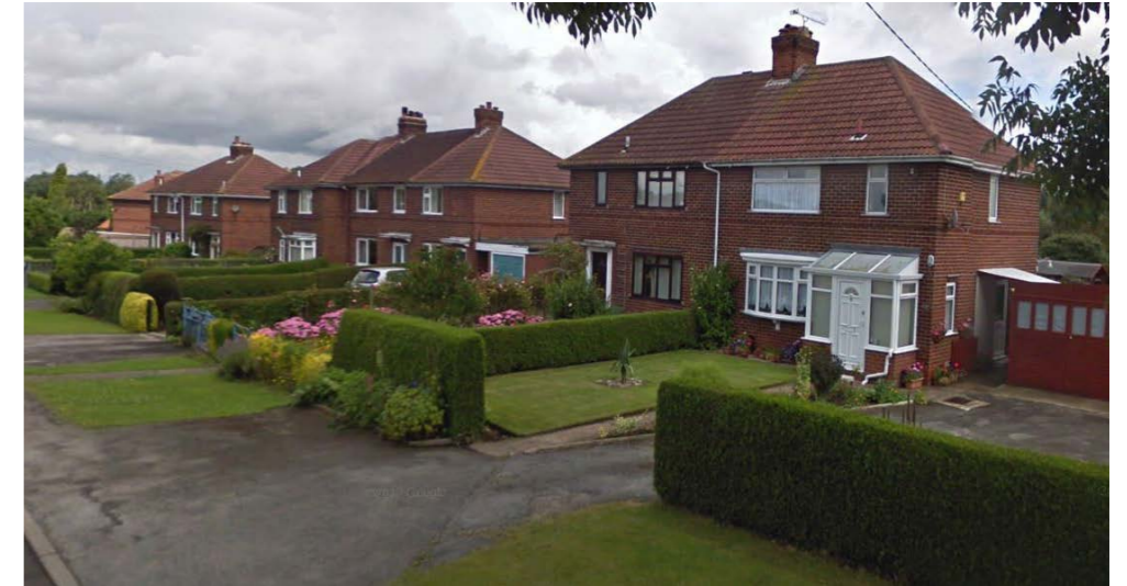
Fig 30: Though pitched roofs are common throughout Treswell, there are several occasions where hipped roofs have been preferred, such as at Cocking Lane, where the adoption of red brick and pantile roofing has helped these buildings fit in despite their more unique form.
