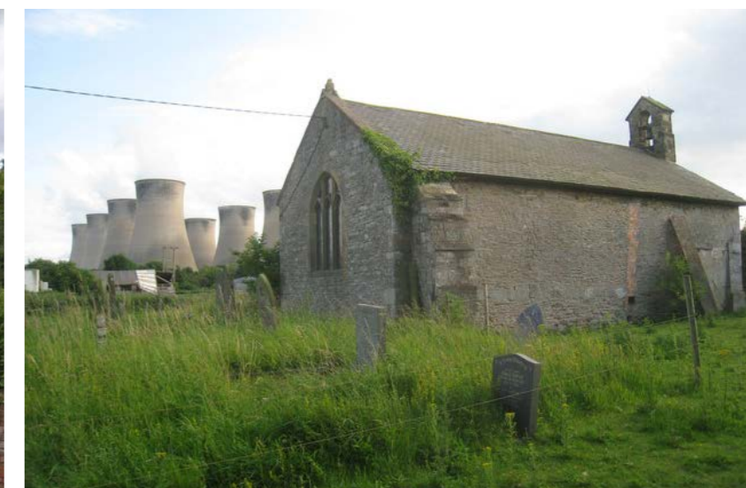
Fig 54: The Church of Holy Trinity is located to the west of the village's central spine within an open and exposed rural landscape. It is constructed of coursed rubble and dressed stone with ashlar quoins and dressings.
