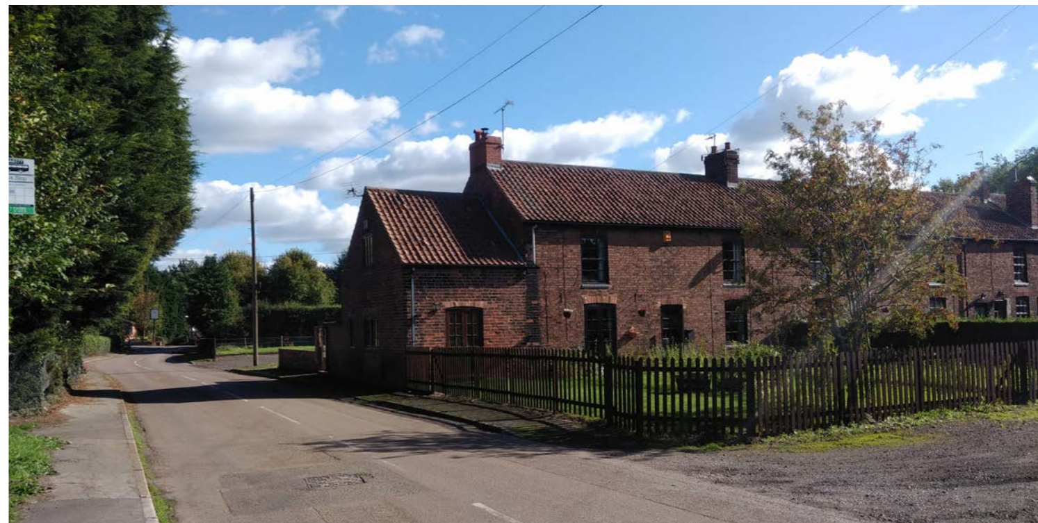
Fig 49: The extensive and handsome red brick facade of May Cottage and Ivy Cottage is one of the most striking buildings at Cottam's southern end. Topped by a pitched clay pantile roof, which is punctuated along the ridge by brick chimney stacks, and with a well-portioned facade with regular window and door arrangements, these cottages represent one of Cottam's finest pieces of local vernacular architecture
