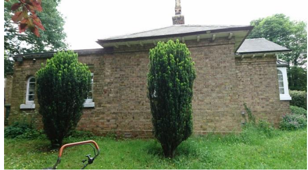
West Lodge, north elevation.
