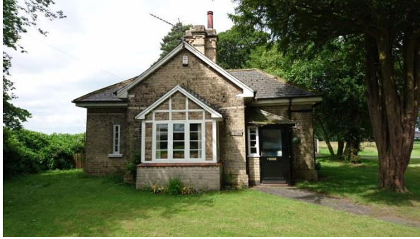
East Lodge, east elevation.
