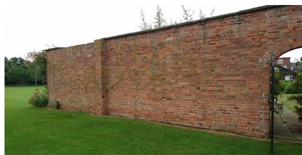
Kitchen garden wall to east of main building.
