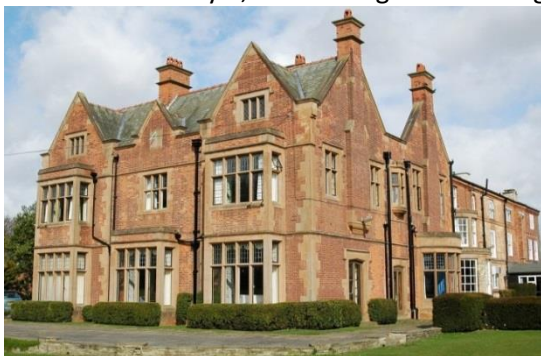
Main façade, viewed from south east.
