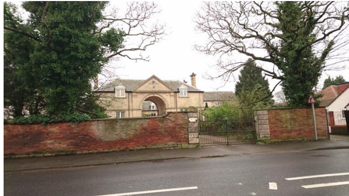
19 th century brick boundary walls across frontage
