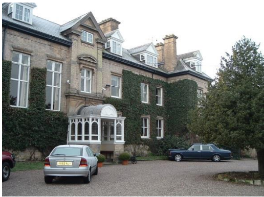
Main façade, 2003 (source: www.wikipedia.org )
