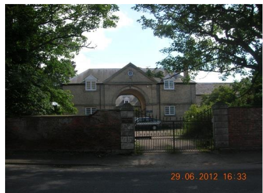
Coach house, wall and entrance gateway
